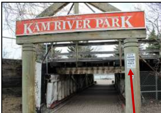
Pedestrian access stays open despite sign
