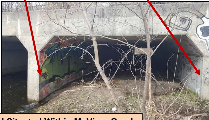
Tunnel Situated Within McVicar Creek
